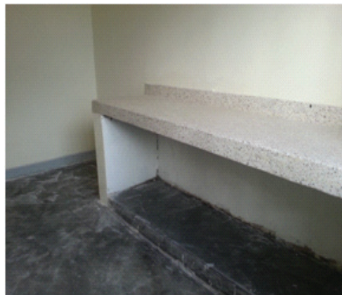
New Work Top at the remodeled laboratory at Nsinze HCIV
