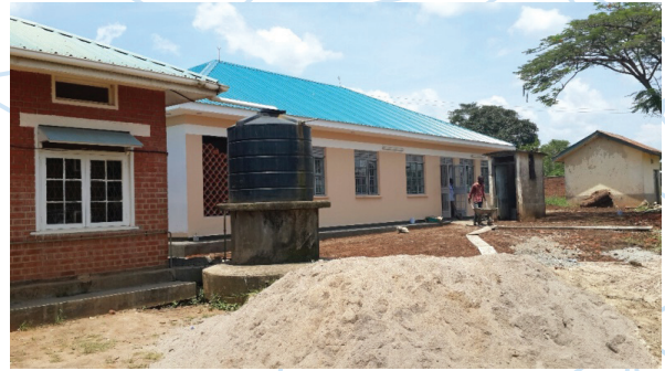
Remodelled laboratory structure at Nsinze HC IV in Namutumba District
